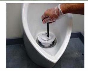
PULL UPWARD ON INSERT TO REMOVE.
