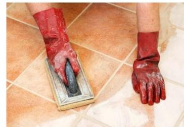
Grout and grout lines may contain additives to provide color, make cleaning easier or extend the life of the grout. Your initial inspection of a job should include examining the grout. Cracks may be present due to movement of the substrate, installation and mixing issues or rarely the quality of the grout itself. Sections of grout that have broken loose due to these cracks can be blasted out by high pressure cleaning.
